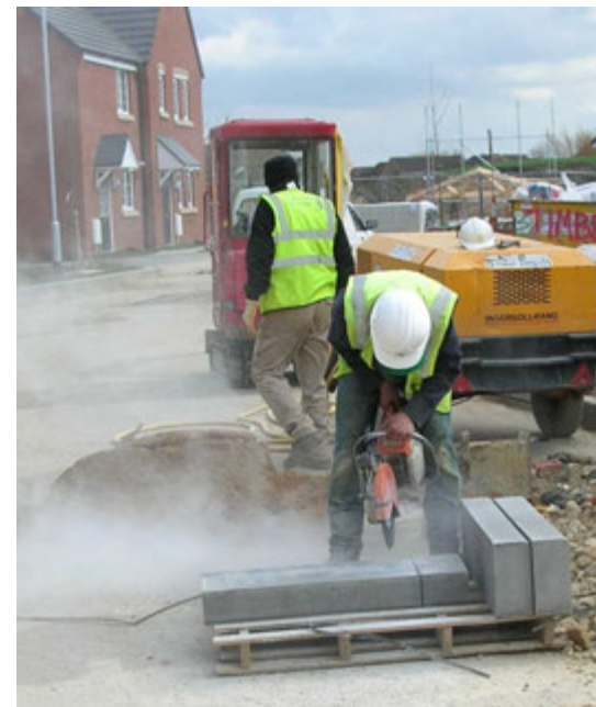
Transportation construction industry concerns about the new OSHA silica exposure regulations include the feasibility of testing within a continually changing jobsite environment, in addition to potential negative effects on overall safety and the health of jobsite workers.
