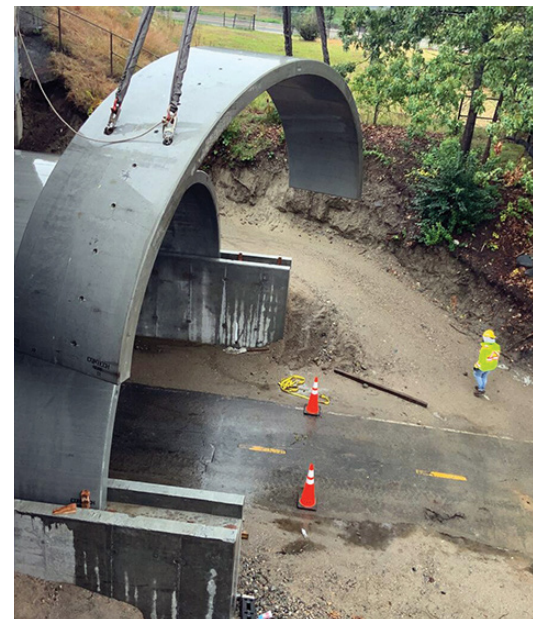
Additional Route 37 Connector work includes paving/resurfacing and precast arch bridge construction.
