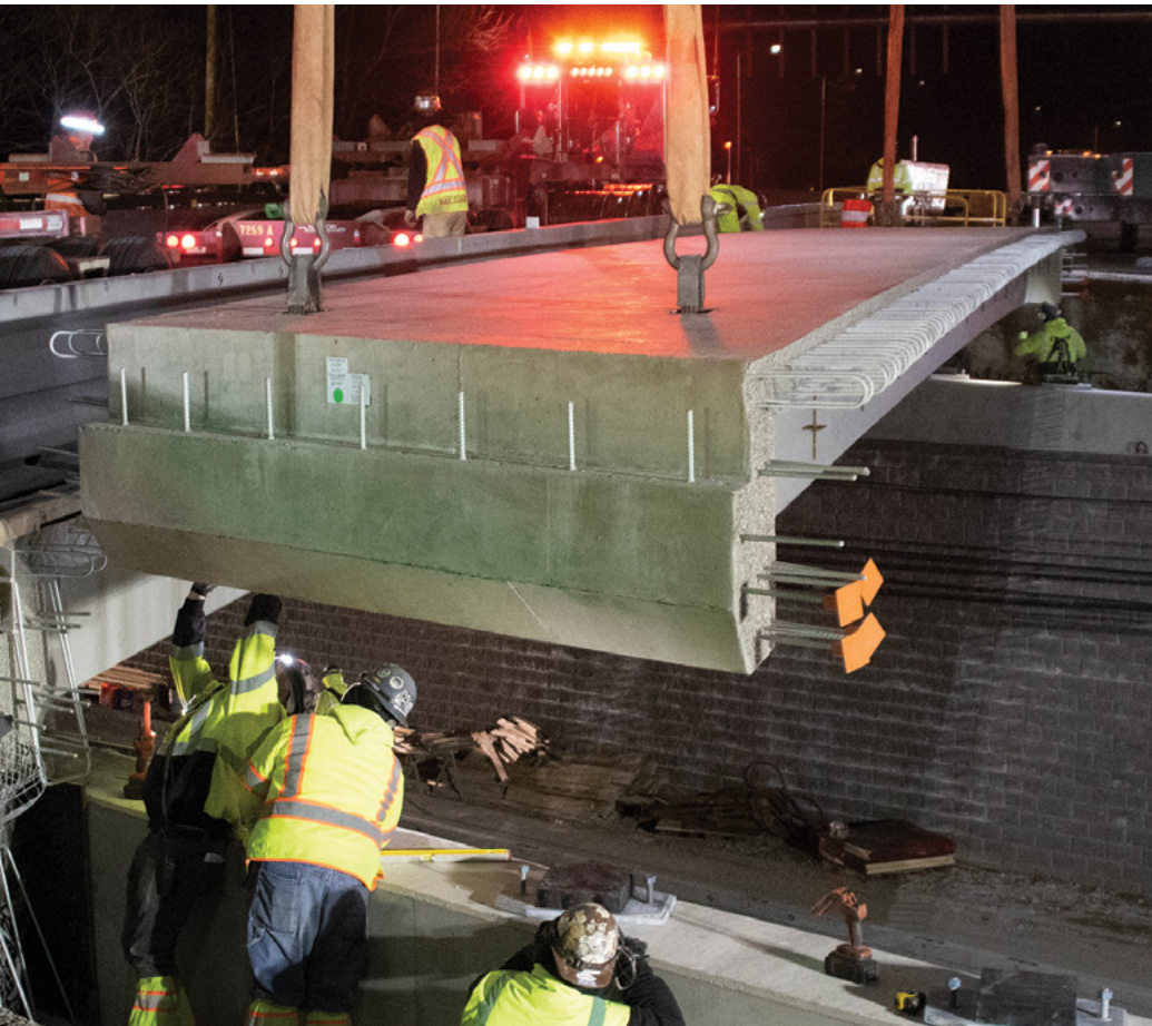
Oaklawn Avenue overpass, Route 37 in Cranston.
