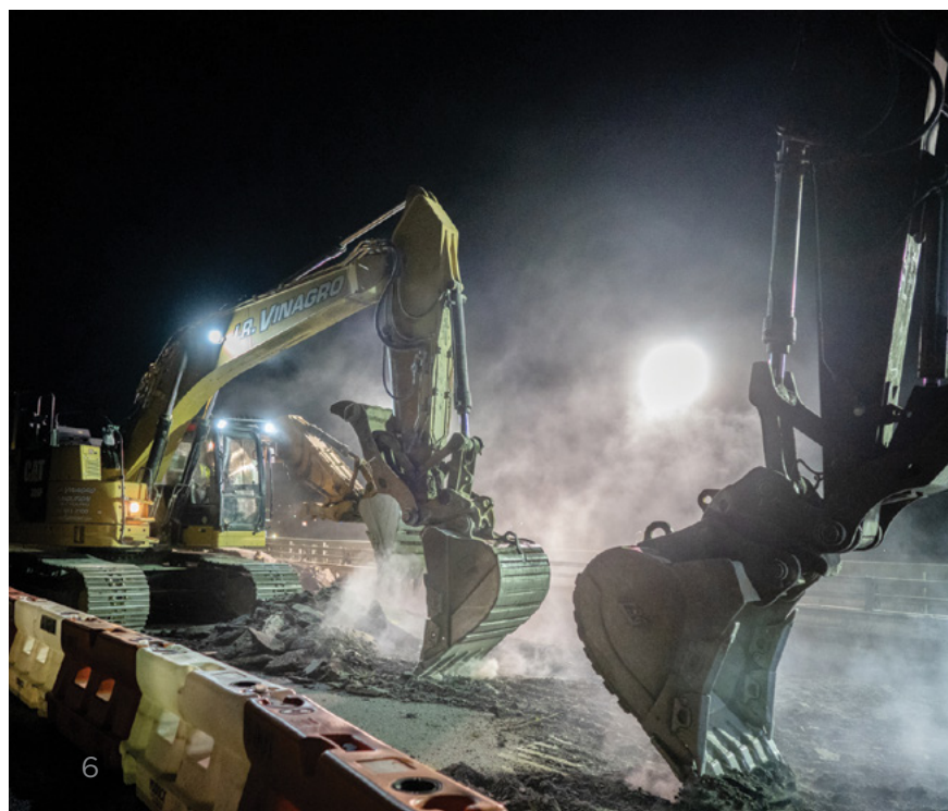
Route 37 eastbound bridge demolition over the Pawtuxet River in Cranston.
