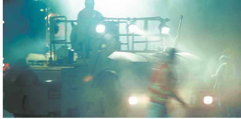
Nighttime paving on Route 146A in North Smithfield.
